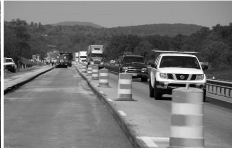
I-81 Pavement Project
