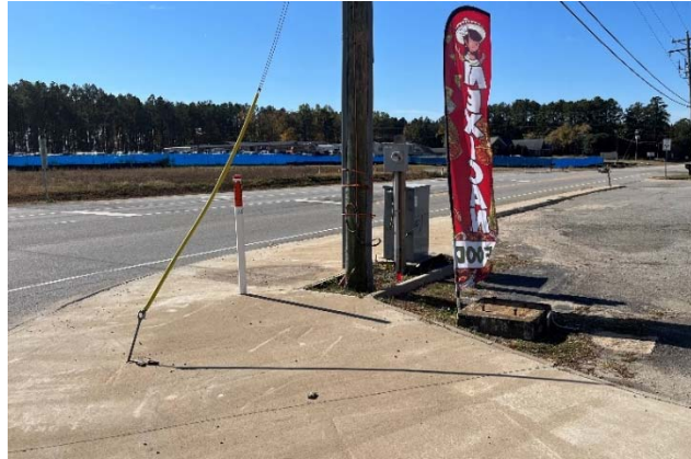
Figure 6 : Northwest Corner of North Mecklenburg Avenue and Tunstall/Union Mill Road (Photo: Toole Design)
