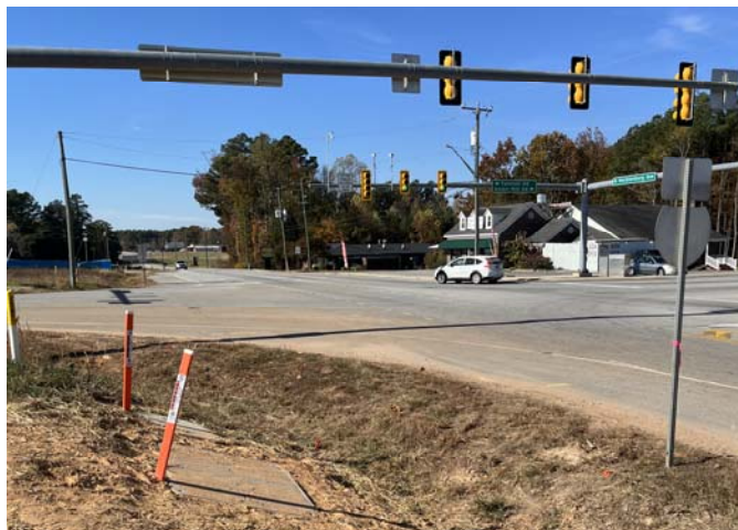
Figure 9: Traffic Signal at North Mecklenburg Avenue and Union Mill/Tunstall Road (Photo: Toole Design)
