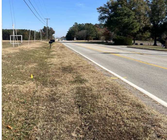
Figure 5: North Mecklenburg Avenue Edge of Roadway (Photo: Toole Design)
