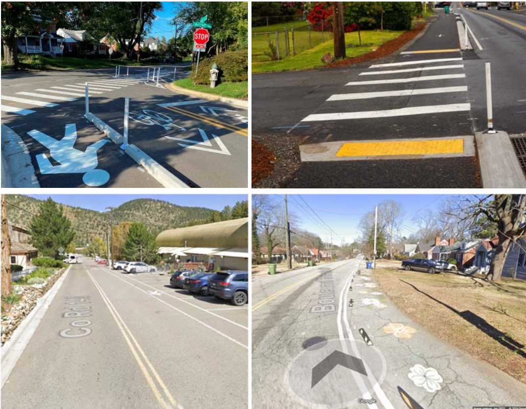
Figure 19 Example Walking Lanes - Clockwise from top left - Silver Spring, MD (Photo: Toole Design), Portland, OR (Photo: Jonathan Maus/Bike Portland), Idaho Springs, CO (Google), Atlanta, GA (Google)
