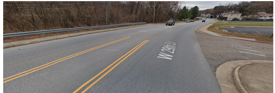
Figure 13 US 60 Lane Reconfiguration, Approaching Orchard Avenue (Source: Google Maps)
