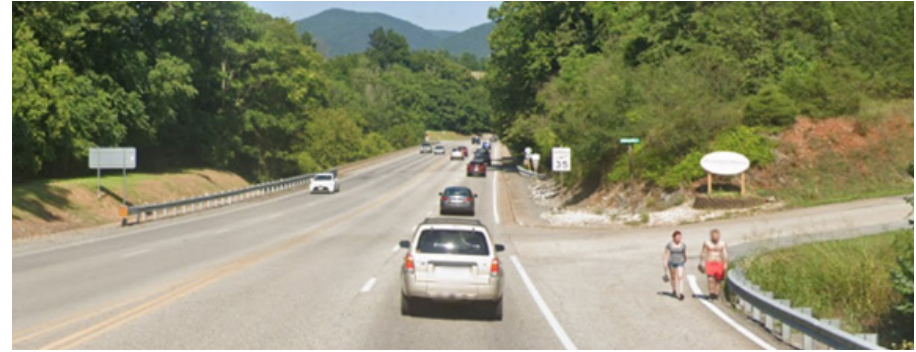
Figure 15 Example of pedestrians walking along the shoulder of US 60 (Source: Google Maps)
