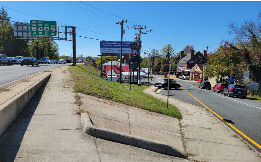
Figure 30: Route 1, left, and West Cambridge Street, right, diverge both horizontally and vertically south of Route 17. West Cambridge Street is a single lane one-way road that is akin to an off-ramp.
