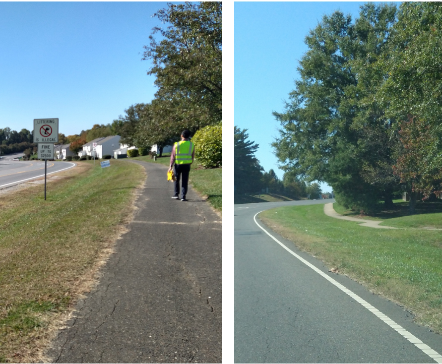
Figure 19: The sidepath along Plantation Drive is narrow for a shared use path, cracked, occasionally concrete, and sometimes merges into the roadway (left: near Truslow Road; right: south of Lichfield Blvd)
