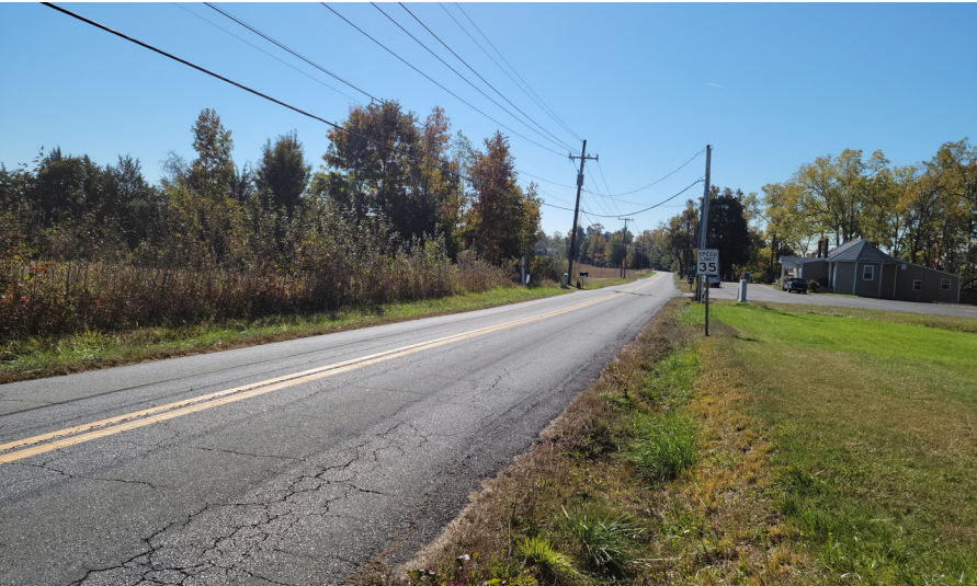
Figure 19: The sidepath along Plantation Drive is narrow for a shared use path, cracked, occasionally concrete, and sometimes merges into the roadway (left: near Truslow Road; right: south of Lichfield Blvd)
