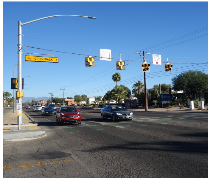
Figure 19. Example of a Pedestrian Hybrid Beacon (PHB), which indicates to drivers when a pedestrian wants to cross (Tuscon, Arizona)
