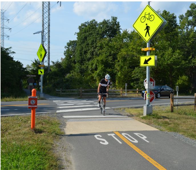
Figure 18. Example of a Rectangular Rapid Flashing Beacon (RRFB) on the W&OD trail in Ashburn, VA
