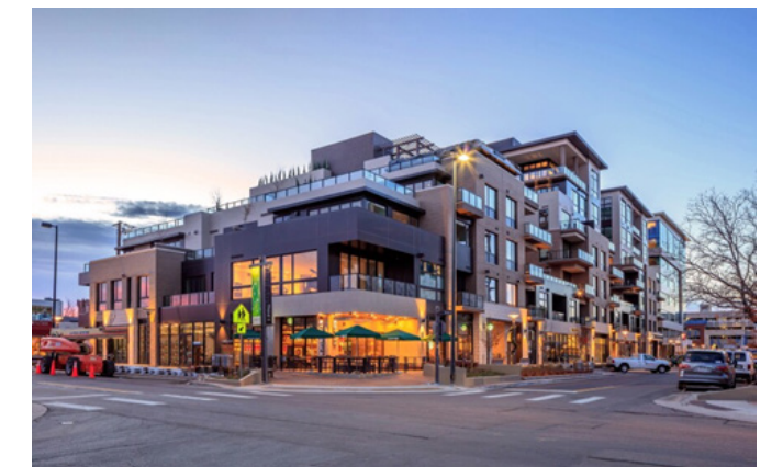
Vertical step-backs reduce the perception of building mass (source: https://cdnassets.hw.net )
